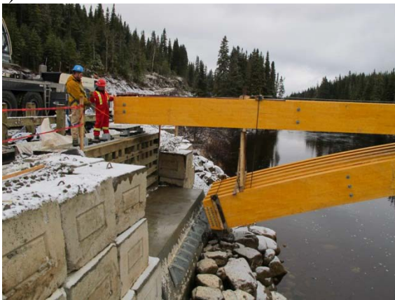
Figure 3. Montmorency Forest Wood Bridge. a) completed project; b) installation of bridge section with a crane; c) installation of bridge section and connectors; d) installation of bridge section and connectors to concrete base; e) installation of connectors to concrete base.
